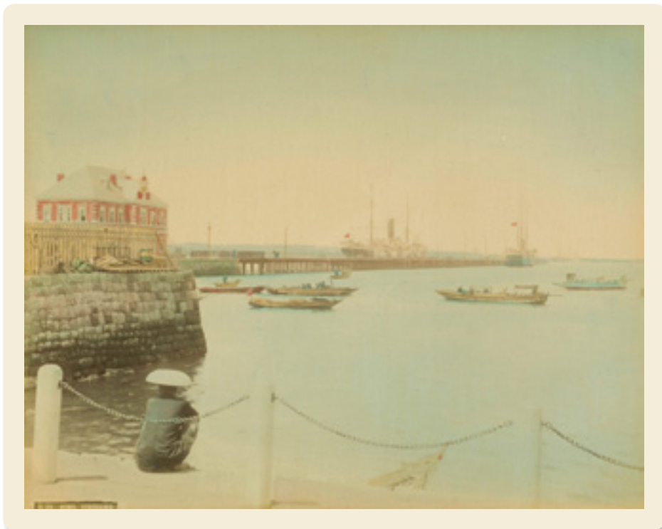
View of pier from Yokohama with two steamships in the background.
